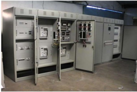
Installed MCC Panels
